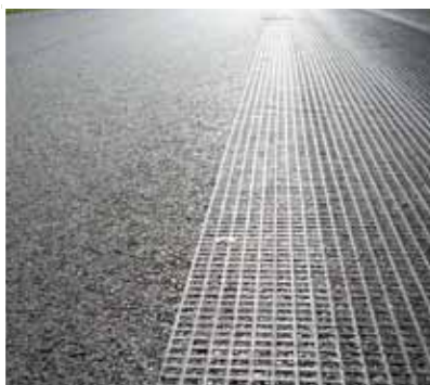
ASPHAGLASS® installation
